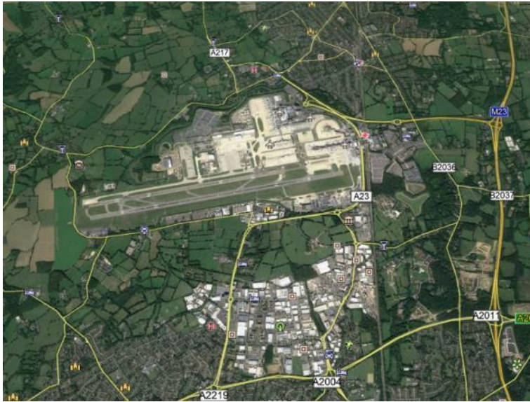
Figure 1 - Aerial view of Gatwick Airport
